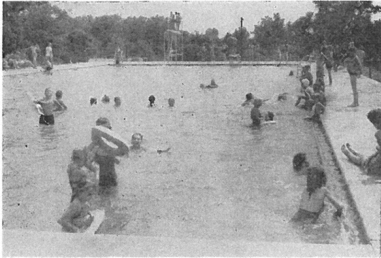
Recently Constructed Municipal Pool
